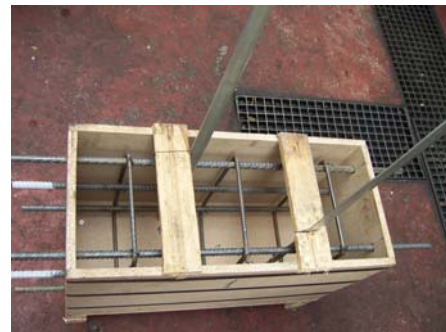
Fig 12: Reinforcement block with various connections
