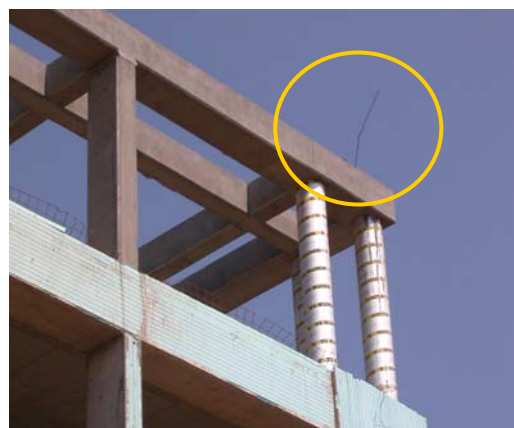
Fig 2: Down conductor installed through the reinforcement
