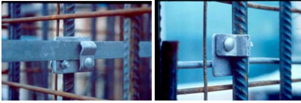
Fig. 3: Approved connectors for connecting LPS conductors with the reinforcement
