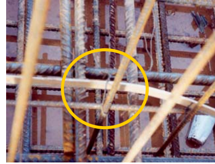
Fig. 5: Non approved connection between earthing tape and reinforcement
